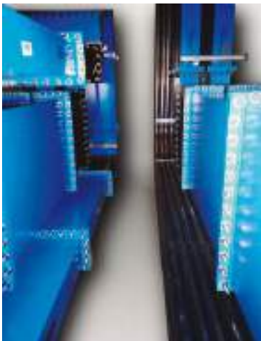
ESS ERIC RF Transmission Line Installation
