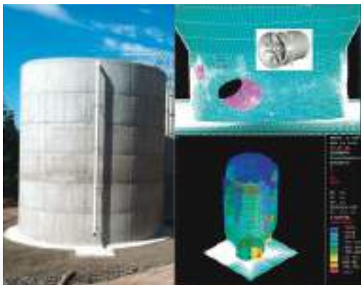
Reinforced concrete tank
