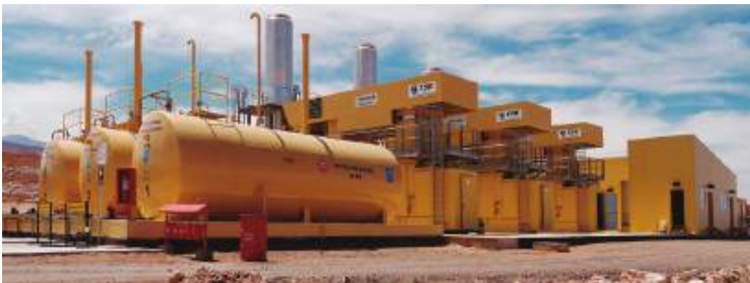
ALMA Multifuel Power Plant (2011)
