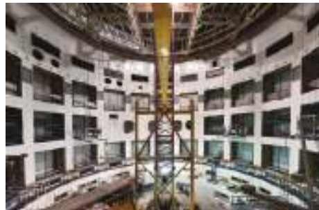
Tokamak Assembly pit_March 19_© ITER Organization-EJF Riche
