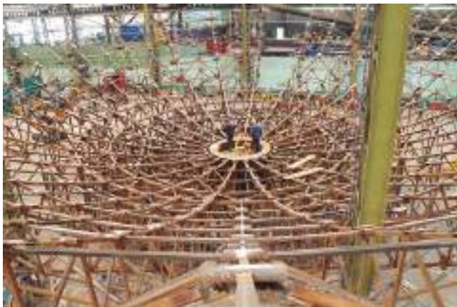
DSN 34m reflector dish back structure shop fabrication
