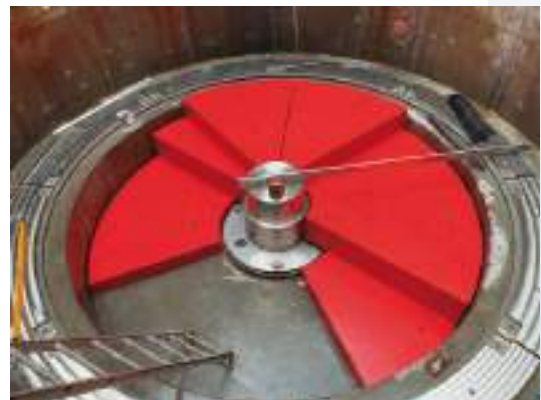
ESS - Vessel support and Ground Shielding
