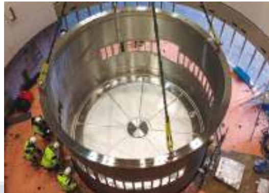
Monolith Vessel Installed in ESS ERIC
