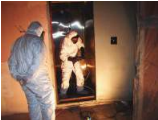
Nuclear Dismantling works
