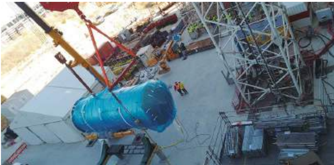
Vessel Installation at ITER
