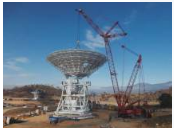
DSN 34m antenna installation in Australia
