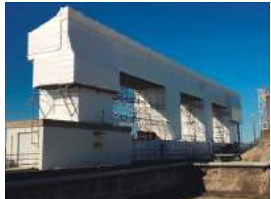
GDES Revanti - Corrosion protection primers, maintenance, paints and coatings. Blayais NPP
