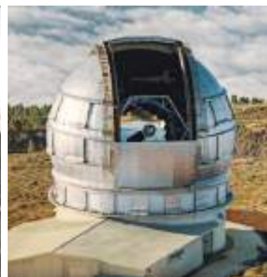
Outside view of Gran Telescopio Canarias
