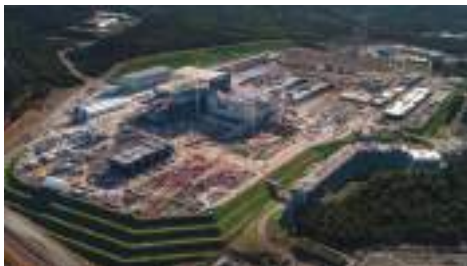
Aerial View_October 19_© ITER Organization-EJF Riche
