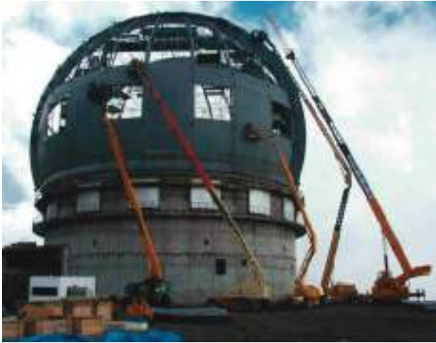
GRANTECAN dome erection
