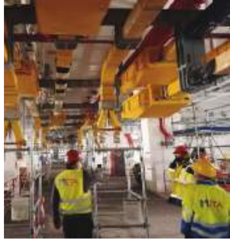
Busbar installation at ITER
