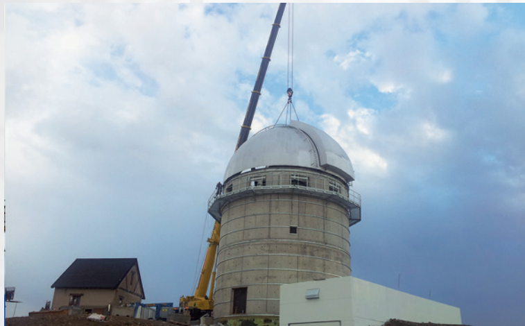
Design & Construction of the Javalambre survey telescope T250 main Dome, 2014
