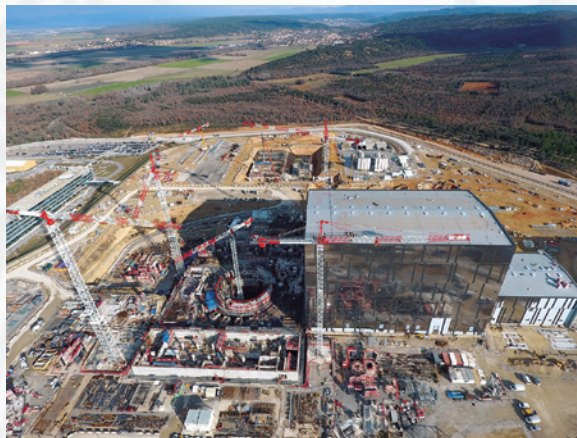
Aerial view ITER
