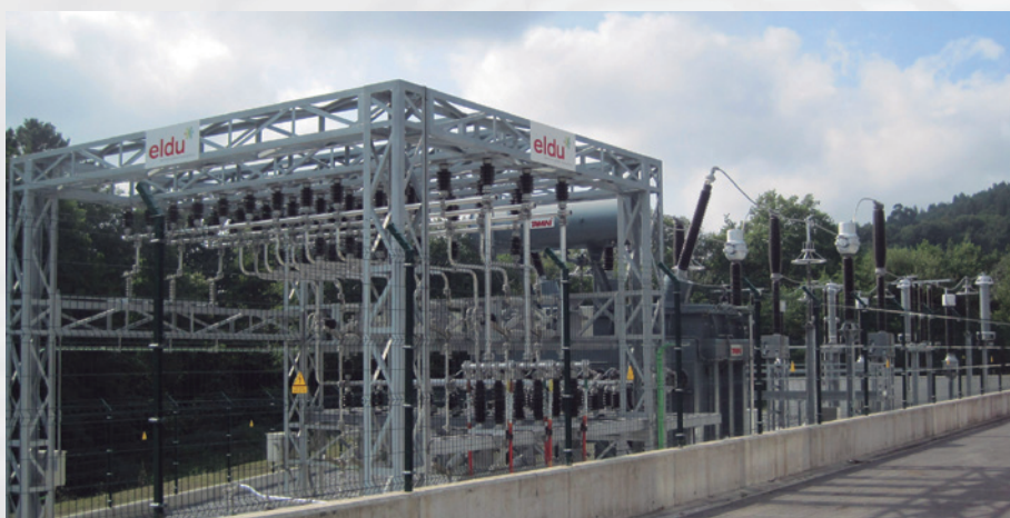
Construction of one 220 KV substation
