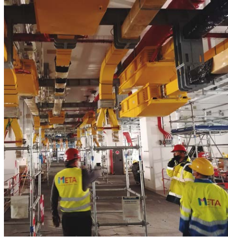
Busbar installation at ITER
