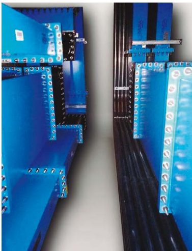
ESS ERIC RF Transmission Line Installation
