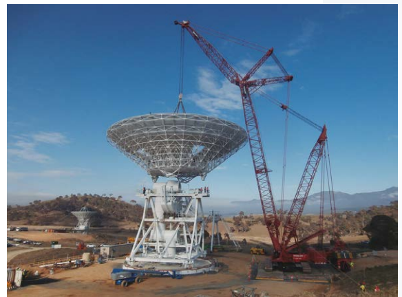
DSN 34m antenna installation in Australia
