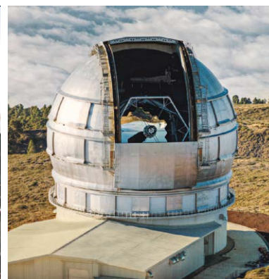
Outside view of Gran Telescopio Canarias
