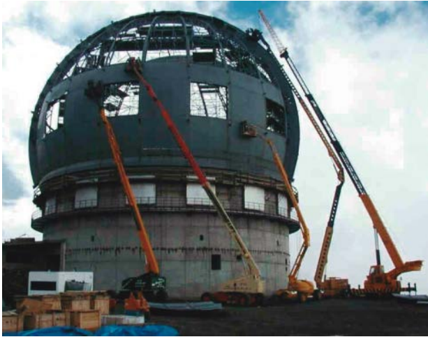
GRANTECAN dome erection
