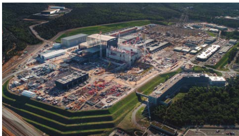
Aerial View_October 19_© ITER Organization-EJF Riche
