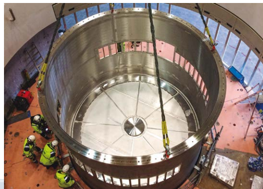
Monolith Vessel Installed in ESS ERIC
