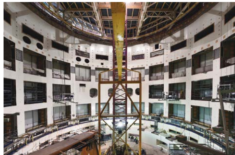
Tokamak Assembly pit_March 19_© ITER Organization-EJF Riche
