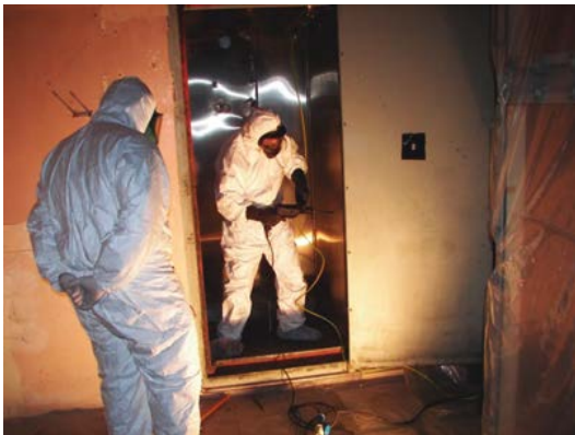
Nuclear Dismantling works
